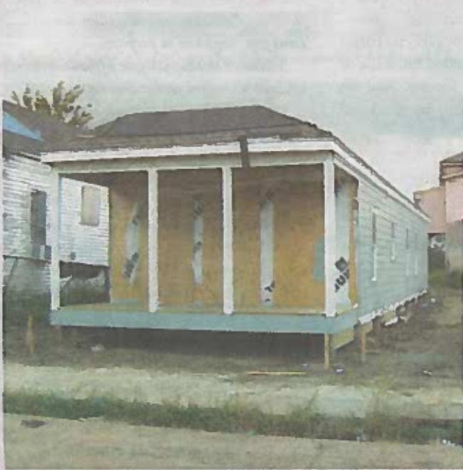
[ABOVE] The first house is in place at 2428 Philip St.
